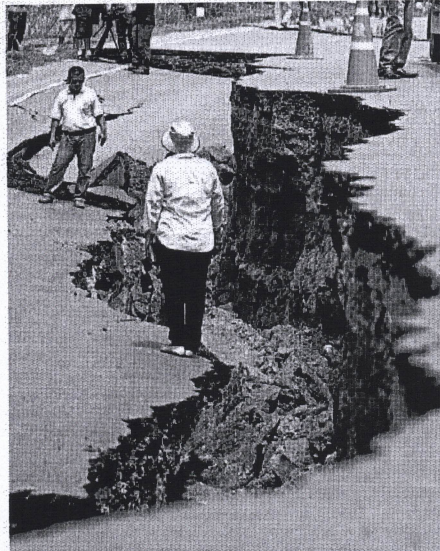
The May 5 earthquake left a gash in this road.
