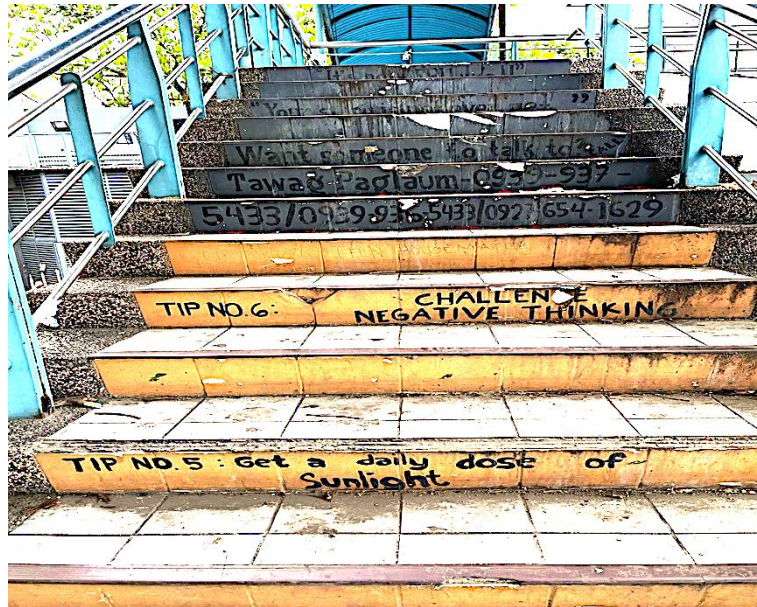
Figure 5 The half landing staircase situated midway up the right-hand staircase (Sidewalk A)
