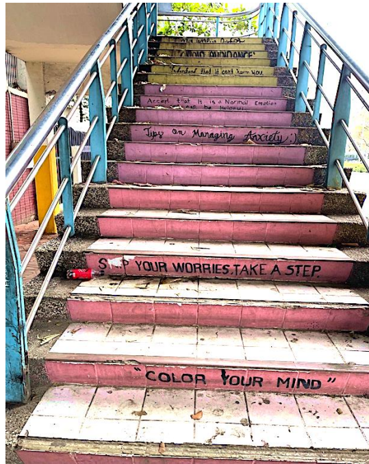
Figure 2 The left-hand main staircase with inscriptions about: “Tips on Managing Anxiety” (Sidewalk A)
